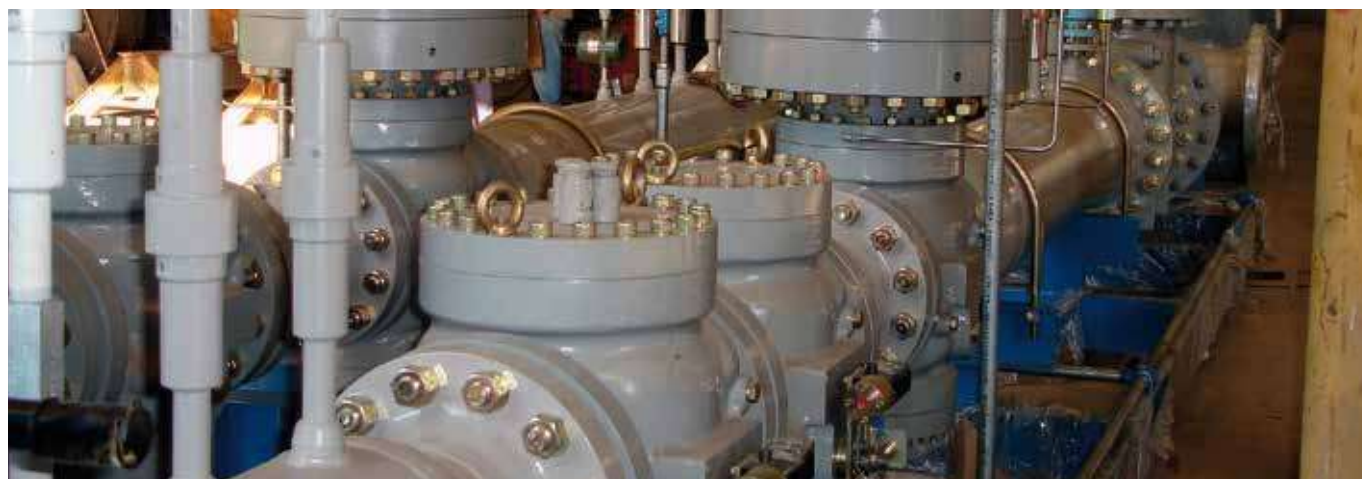
TA-956 FC and SSV DN200 ANSI 600 Customer: Bemco project in Marib, Yemen
