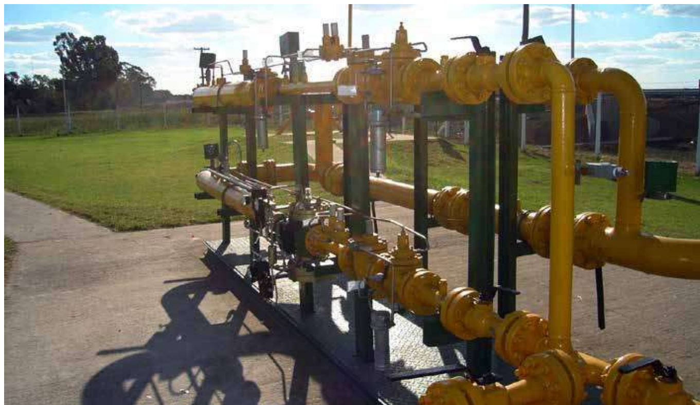
TA-956 DFO+FC+SSV DN80 ANSI 600 Customer: EMGASUD Project: Buenos Aires, Argentina
